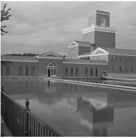
THE WATERWORKS ON CONDUIT ROAD, AKA THE DALECARLIA AQUADUCT, CIRCA 1940.
