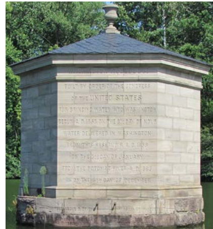
THE OCTAGONAL STONE SLUICE TOWER IN DALECARLIA RESERVOIR, WHICH ORIGINALLY CONTROLLED THE OUTFLOW INTO THE CITY WATER SYSTEM
