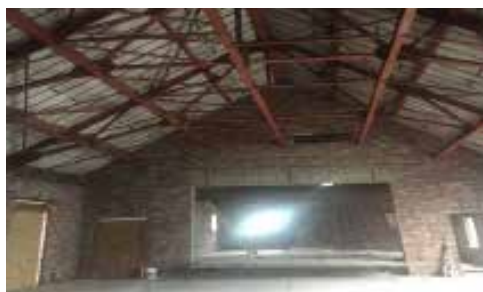
INTERIOR DEMO PROGRESS
